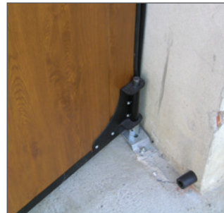
Bottom fixing plate with lateral adjustment
