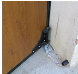
Bottom fixing plate with lateral adjustment
